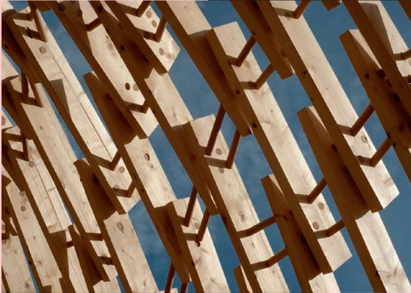
Timber Dowel Assemblies, Gradual Assemblies project; constructive system using oriented dowels to form a spatial joint. A timber-only construction combining a digital fabrication approach with computational geometry and manual craft. © Martina Cirese
